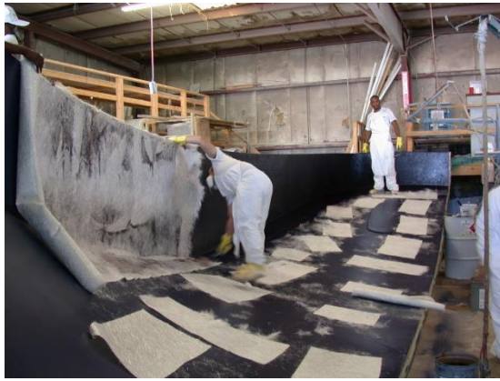
Fig.6.2 Localized fabrication with GFRP in boats.
