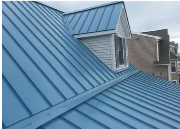
Fig 1.14: Metal roofing sheets
