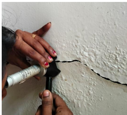
Figure 6.5: Crack width measuring using Elcometer
