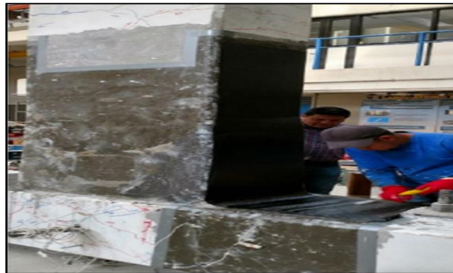
Figure 1.4 Fixing CFRP sheets to beam-column joint (Source: Rodríguez et al., 2021)
