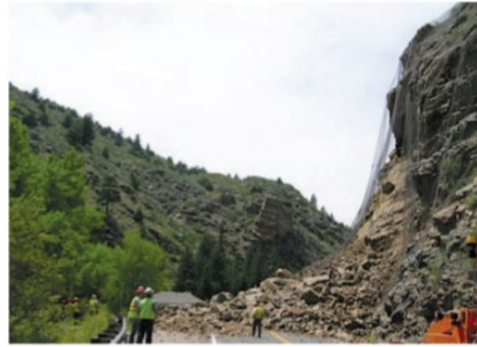
Figure 2.3 rockfall /slide clear at Creek Canyon, Colorado, USA, in 2005
