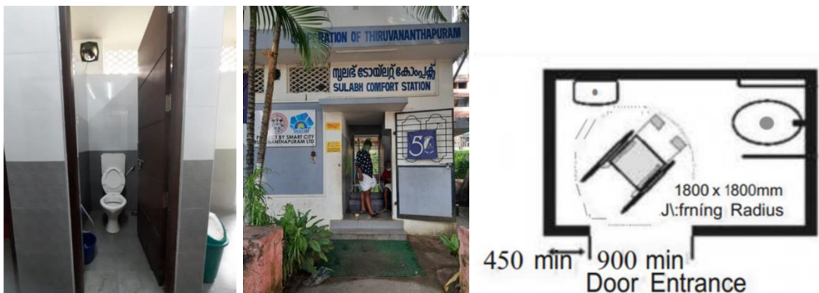
Figure 32 Public toilets retrofitting
