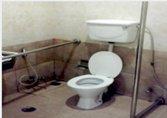
TOILETS FOR PERSONS WITH DISABILITIES
