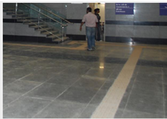
TACTILE PATHS FOR THE VISUALLY IMPAIRED
