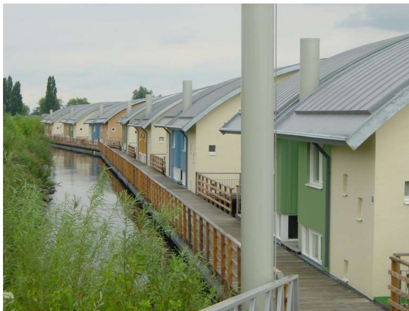
Figure 14 - Amphibious housing - mooring posts (Maasbommel)
