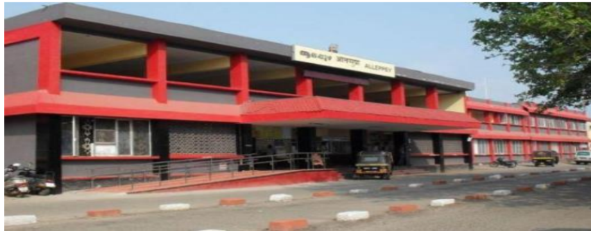
Fig 4.3 Alappuzha Railway Station
