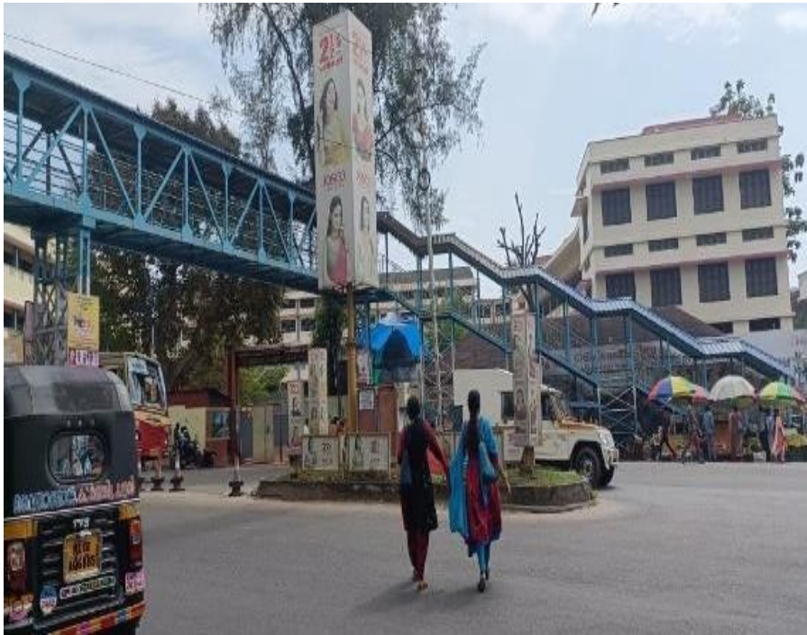
Figure 3.3 Footbridge in Convent Junction
