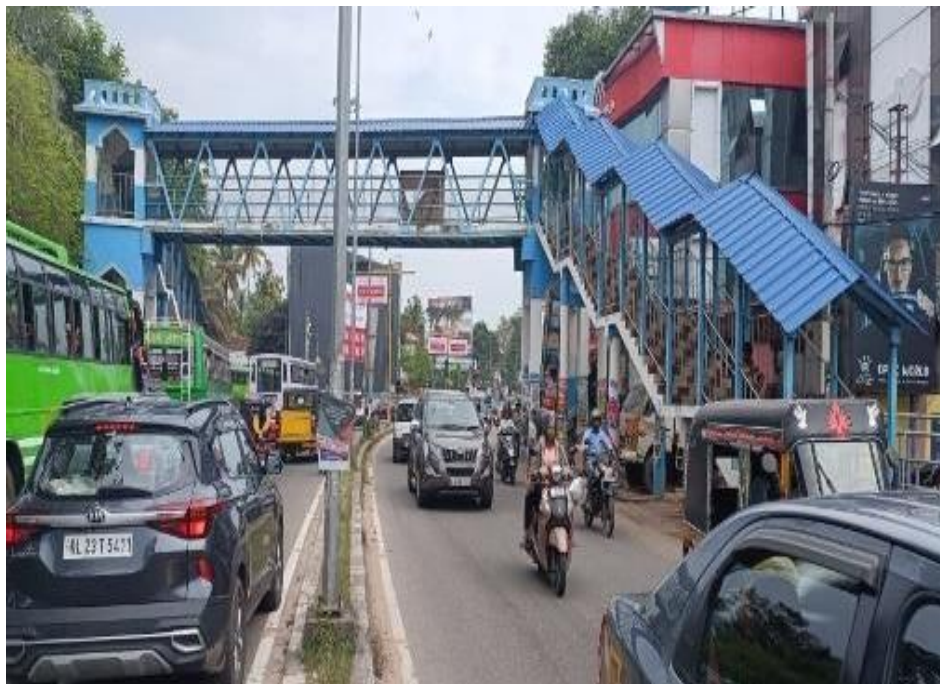
Figure 3.2 Footbridge in High School Junction
