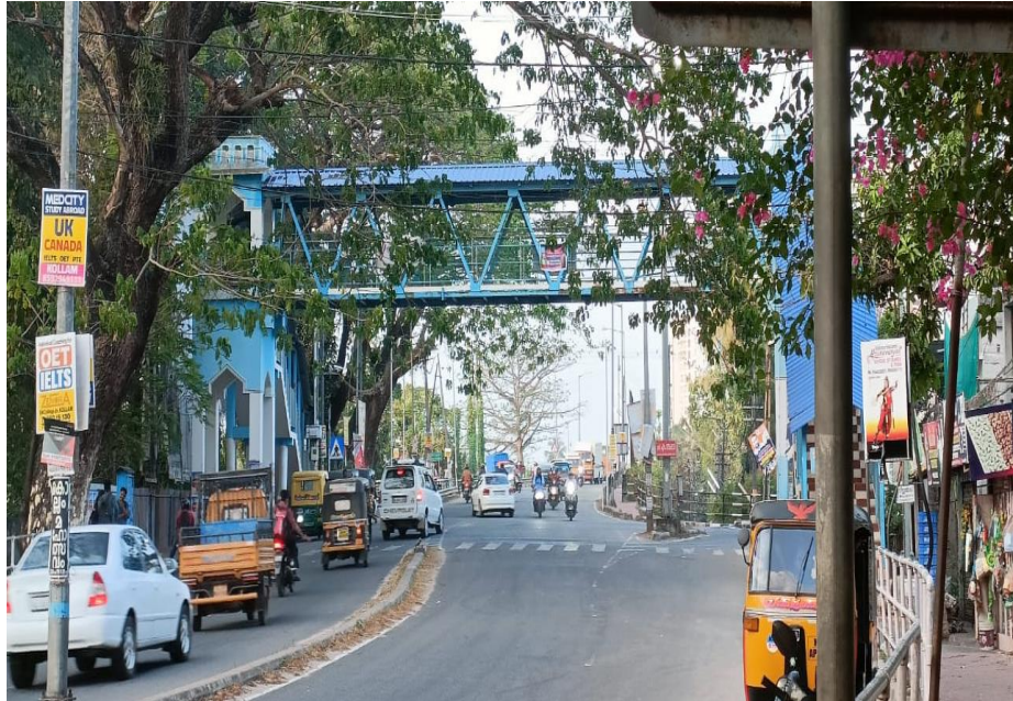
Figure 3.4 Footbridge in Chemmanmukk
