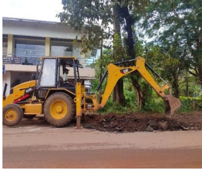
Figure 3.11 Collection of RAP Materials from Anayadi Highway Work
