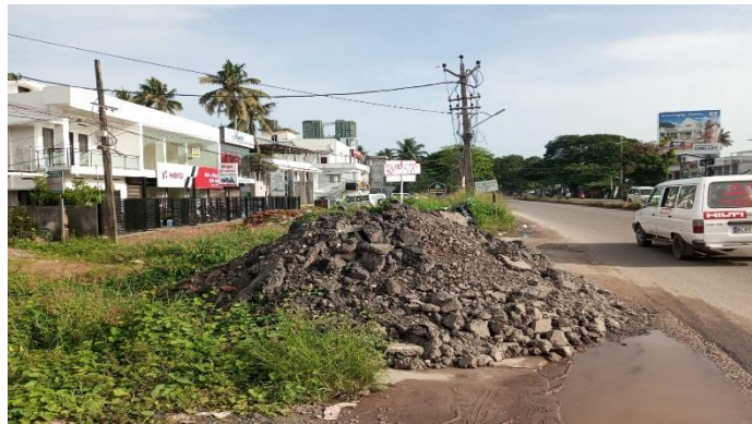
Figure 1.1 Stockpiled RAP Materials- Kazhakootam Elevated Highway Works
