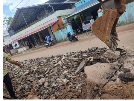
Figure 3.11 Collection of RAP Materials from Anayadi Highway Work
