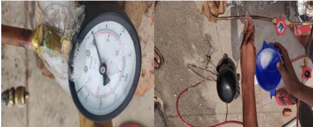
Fig. 6.10: Photograph of leakage testing of the system
