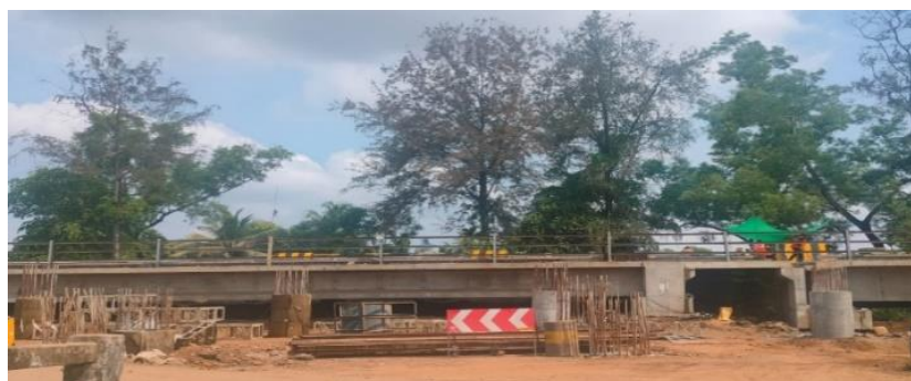
Figure 4:36 : Ongoing construction of AC road in Kuttanad taluk
