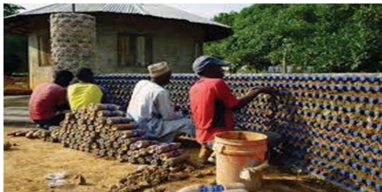
Figure 5:22: Brick bottle technology
