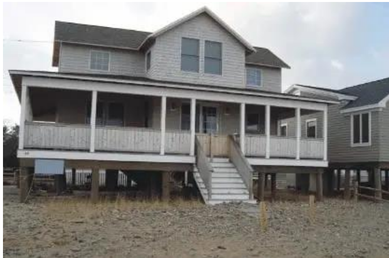
Figure6.7 Flood resistant structures
