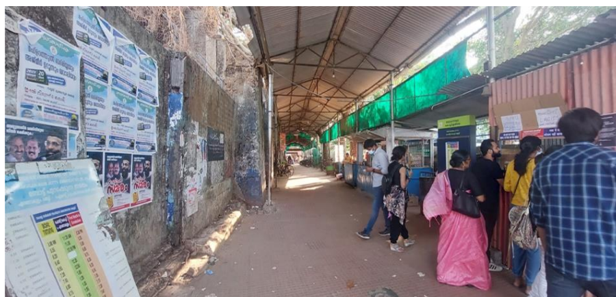
Figure 8. 10 Existing condition of Boat Jetty
