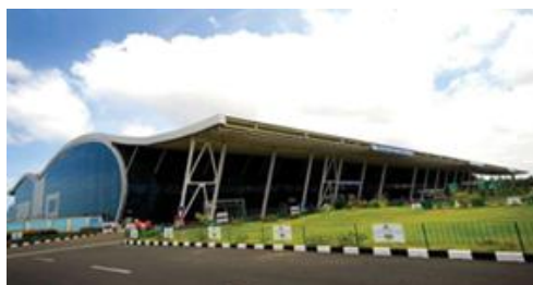
Figure 3. 13 Thiruvananthapuram international airport
