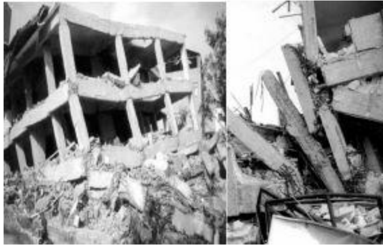
Figure 1.1 Typical beam-column joint failures (1999 Turkey Earthquake)
