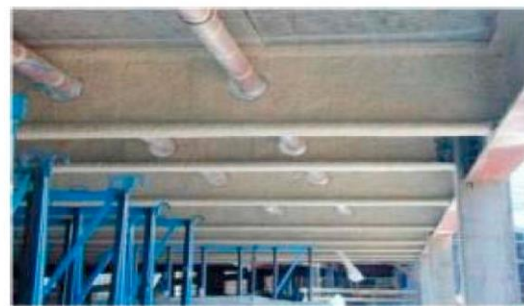
Figure 1.1 Transvers beam opening in beam column joint
