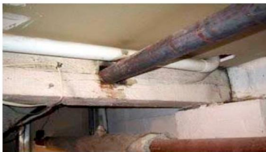
Figure 1.1 Transvers beam opening in beam column joint
