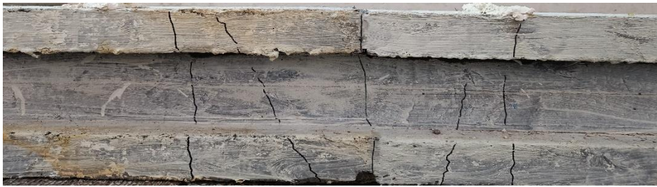
Figure 5.6 Crack pattern of SC ECC ferrocement I beam
