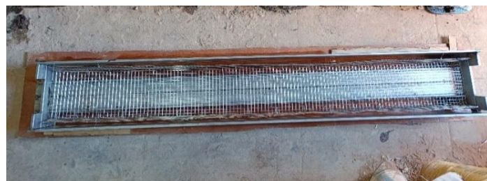
Figure 4.22 Placing of reinforcement mesh in the mould
